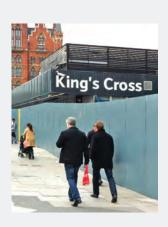
Network Rail approved **Secure Hoard™** has been designed for quick and easy installation by using Blok N Mesh's patent pending H Section arrangement. Flat face panels allow the use of graphics and advertising on the hoarding panels. Blok N Mesh are able to provide you site-specific wind calculations and crowd calculations for your site, which will indicate whether you require the back-stay arrangement every 1.2 meters or 2.4 metres.
