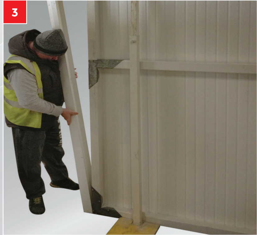
Place H Section on the Panel.
