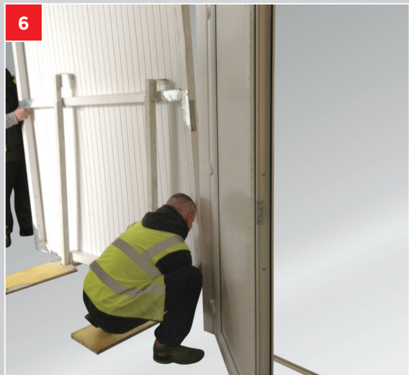
Place Upstands in place as above and slide Panel into H Section.
