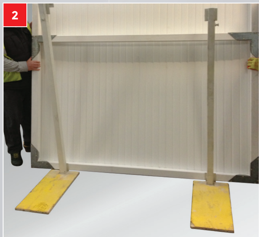
Place Panel into Upstands.
