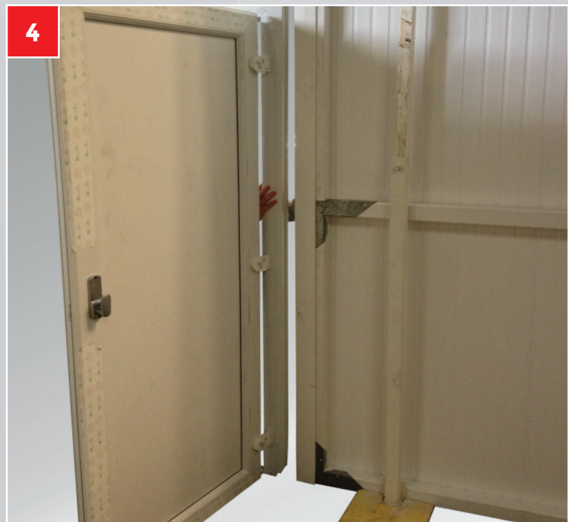
Place Door into H Section – Leave door open.
